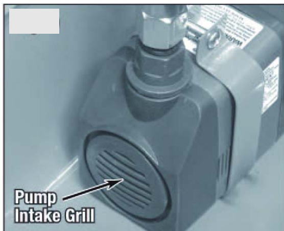
Fig. 12: Cleaning the pump grille
