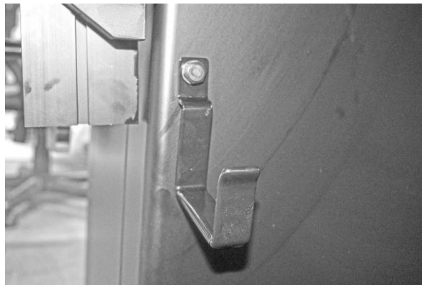
Fence Hook Installation
