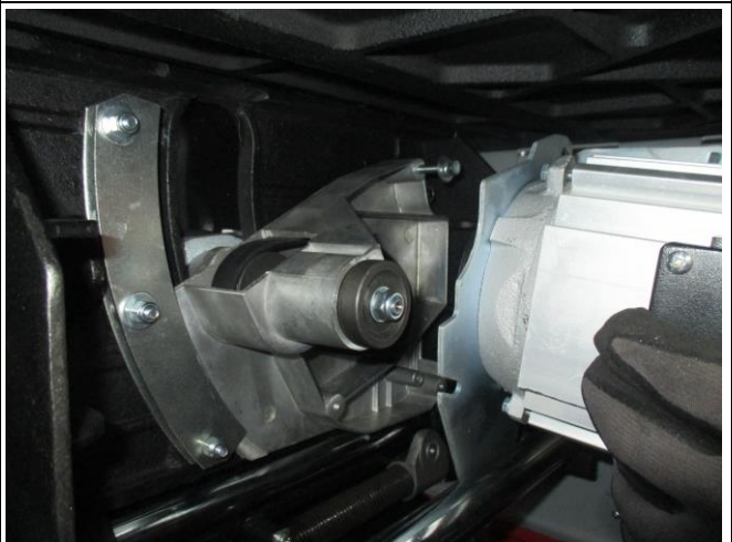
The motor can now be removed and stored with the wiring on the ground.
